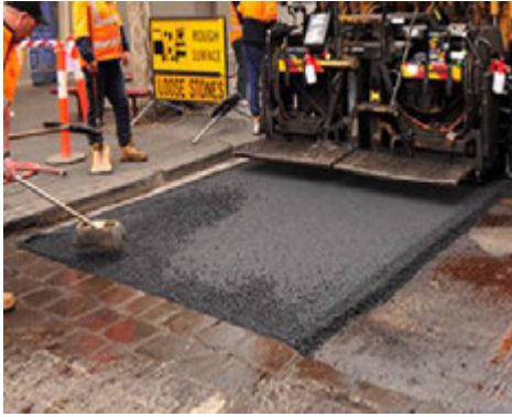
Around 100 tonnes of recycled glass and plastic have been used in a road resurfacing project in Melbourne's City of Yarra.
