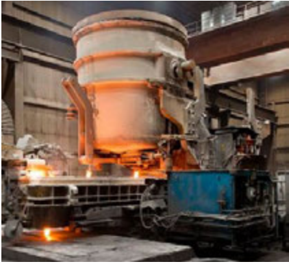
Bottom Taping of Steel Ladle with High Tech. Refractory Silde Gates.
